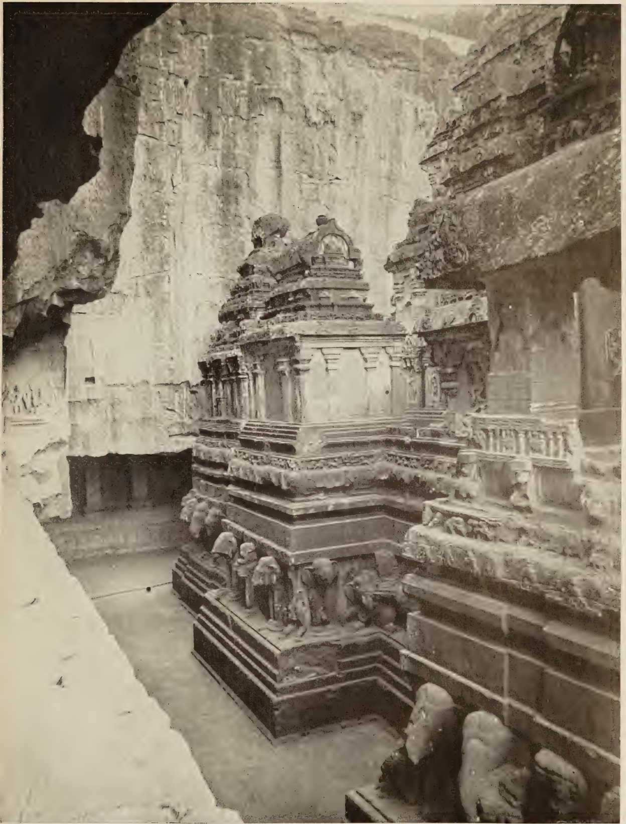
END VIEW OF THE KAILASA, SHOWING TWO OF ITS SHRINES
